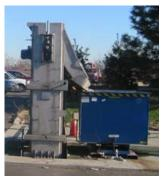
For many years the pump station had manual screens located below grade. The screens required manual raking down in a dirty confined space, an area that flooded during every major rain event. According to information from our rep in the area, John Corkery with Pumping Services, "the screens failed numerous times and the pump station was rebuilt once as a result of severe flooding before the Headworks® screens were installed.'
