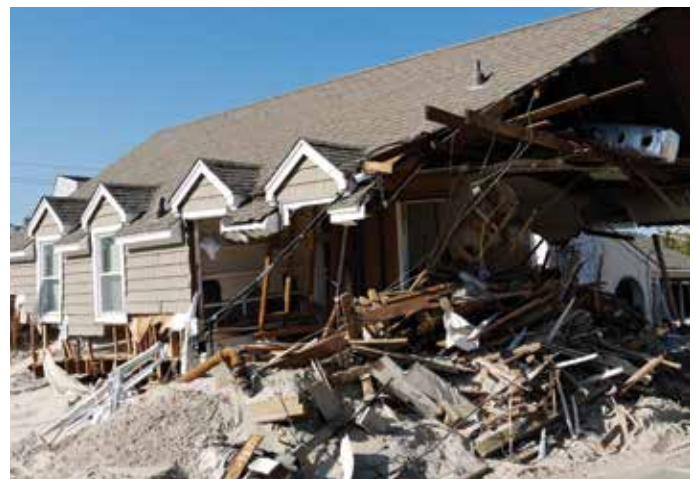
Destruction from Superstorm Sandy in Mantoloking, NJ.
