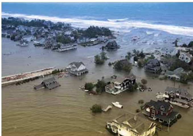
Route 35 after Superstorm Sandy made landfall.
