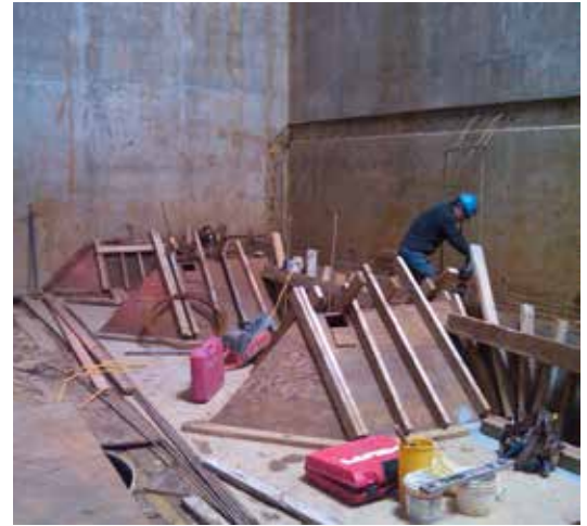
Construction of Sump
