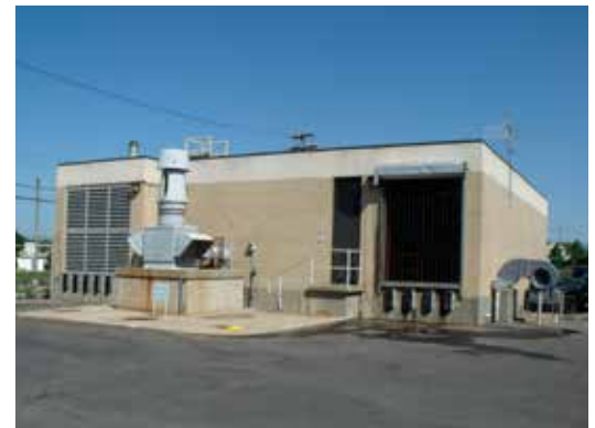
Outside view of Baltic Avenue pump station.
