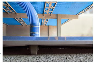
SedVac can easily be retrofitted into existing plants with minimal work to the basin. Swept width typically spans a width of 24', and because of its springloaded chassis and traction drive, has covered a length of up to 330'. Considerations to the length covered by one unit include the speed at which it is run and the number of cleaning cycles it will have to perform in a day.
