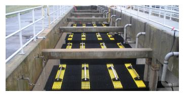
The submerged fixed-film or fixed-bed bioreactor (FBBR) system increases treatment capacity and efficiency by adding to the biomass inventory of the system as bacteria grow on the surface of the media. The unique design of Brentwood's AccuFAS system combines aeration, proprietary distribution media, and vertical flow media to create an airlift pumping mechanism that not only provides sufficient substrate and oxygen to the bacteria in the biofilm, but also maintains thin film thicknesses.
