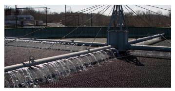
Trickling filters offer a simple, cost-effective, energy-efficient treatment solution. With more than 500 trickling filter installations worldwide, Brentwood's media and components have been optimized to guarantee the best performance for any application. By maximizing surface area in a given volume while maintaining the structural integrity required for deep towers, Brentwood's structured-sheet media provides an ideal environment for microorganism growth.
